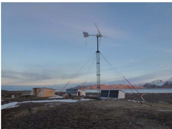
The Corbel Station
