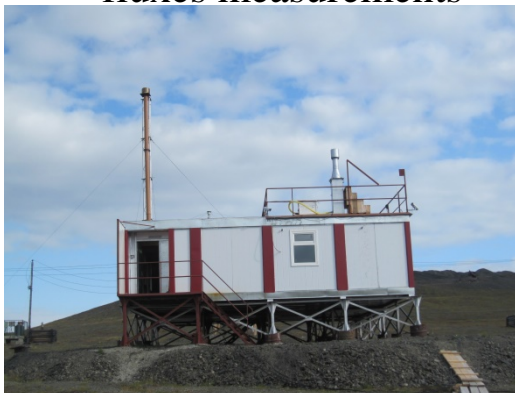
Clean air facility
