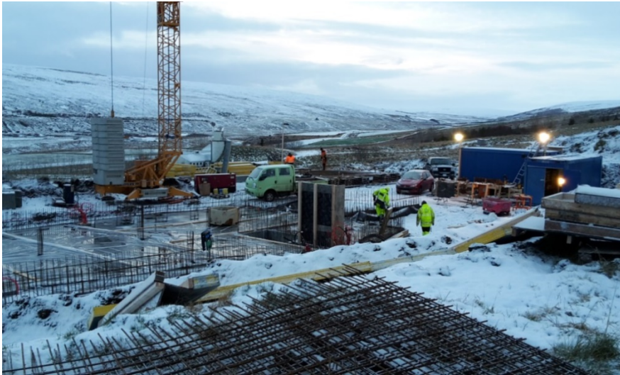
New Aurora Observatory under construction (started from May 2015)
