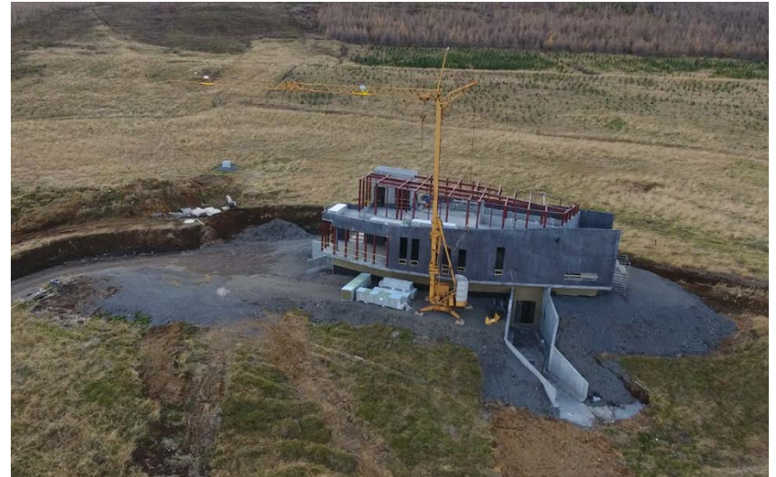
New Aurora Observatory under construction (Jan, 2016)
